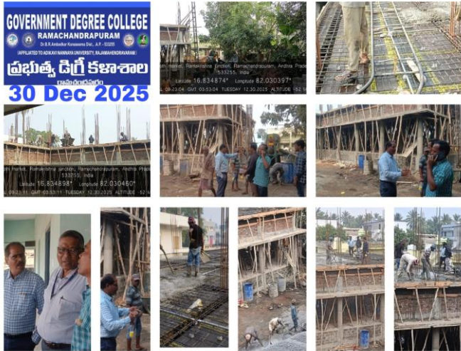
Monitoring of construction of Ground Floor Slab Under PMUSHA
