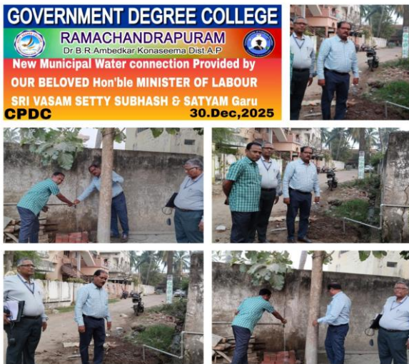
Municipal Water Connection at GDC, Ramachandrapuram
